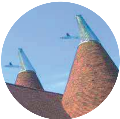
OAST HOUSE CONICAL ROOF- COWL AND VANE DETAIL
