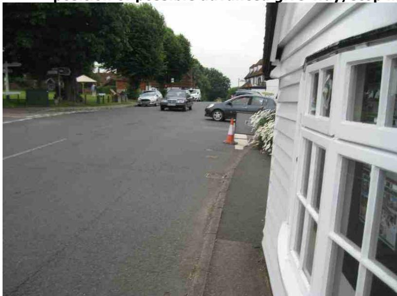
The added benefit of the lining proposals is that the lay-by adjacent to the shops is deepened which would allow vehicles that park here without encroaching into the main carriageway area as existing. The budget sum of these white lining proposals which would also require road studs to be relocated is about £3,000.
