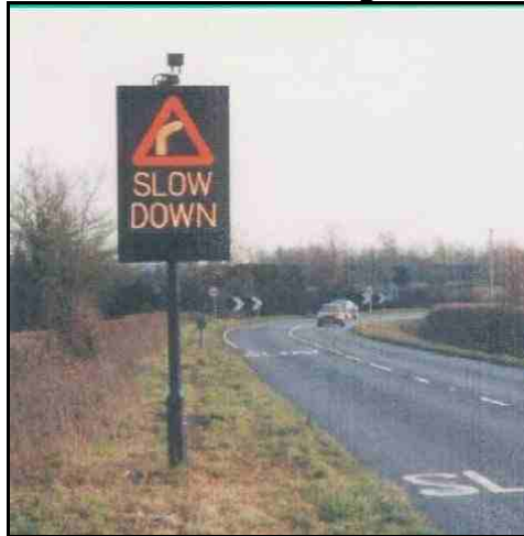
Photo 2: Example of Vehicle Activated Sign – ‘Bend Ahead’ Warning Sign
