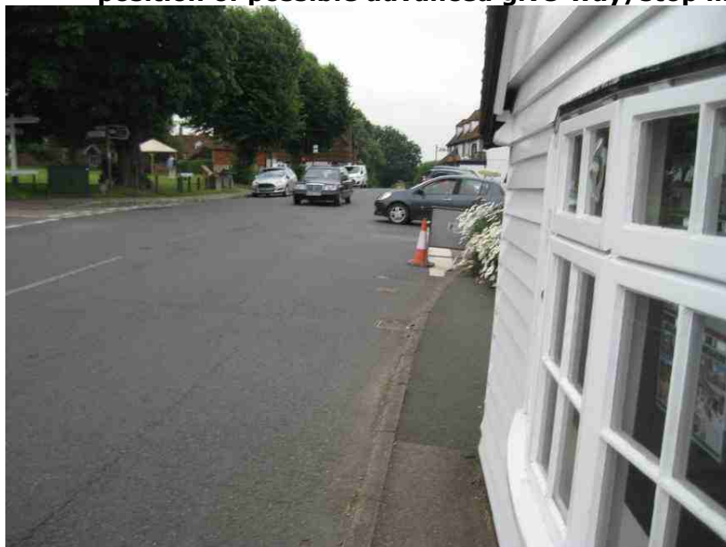
Photo 3: Brenchley Rd looking east to crossroads junction with exiting car at position of possible advanced give-way/stop lines
